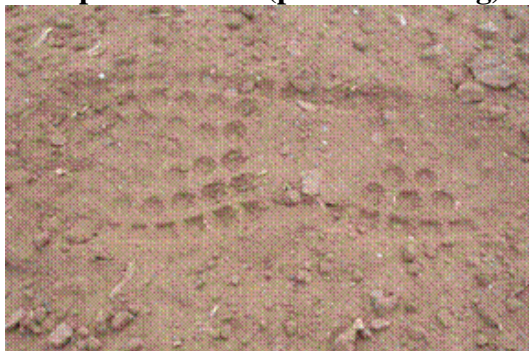
Proper firmness (prior to seeding)
